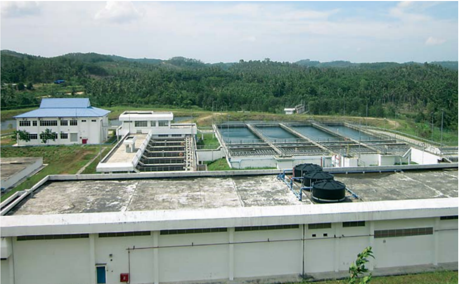
Kudat 60MLD Water Treatment Plant
