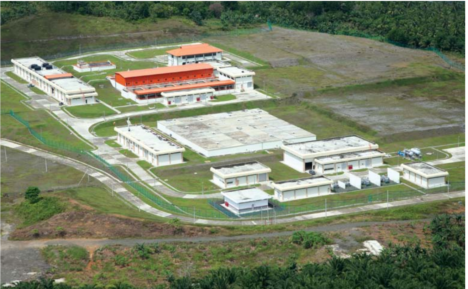
Sandakan 125MLD Water Treatment Plant
