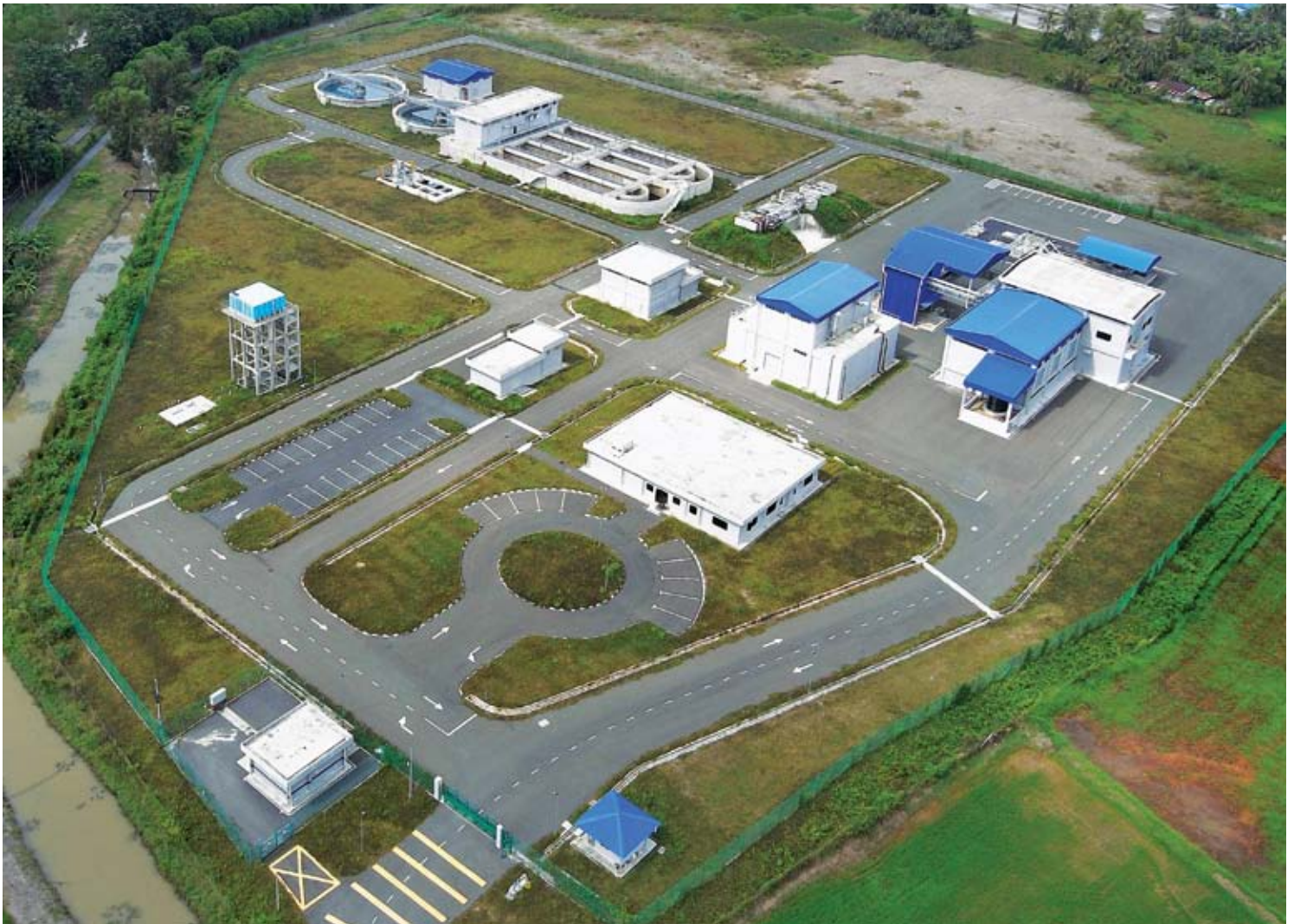
Sungai Udang Centralised Sewage Treatment Plant (300,000 PE)
