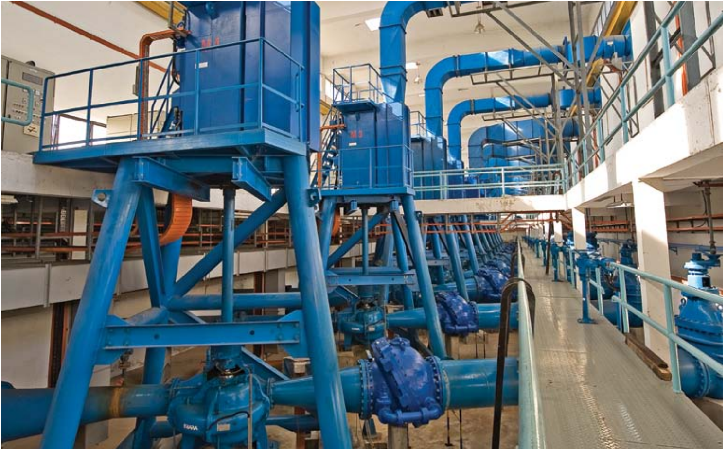
Sg. Selangor Water Supply Scheme Phase 2 Package 4 (2 x 142MLD 1540kW and 3 x 72MLD 810kW treated water pumpsets)
