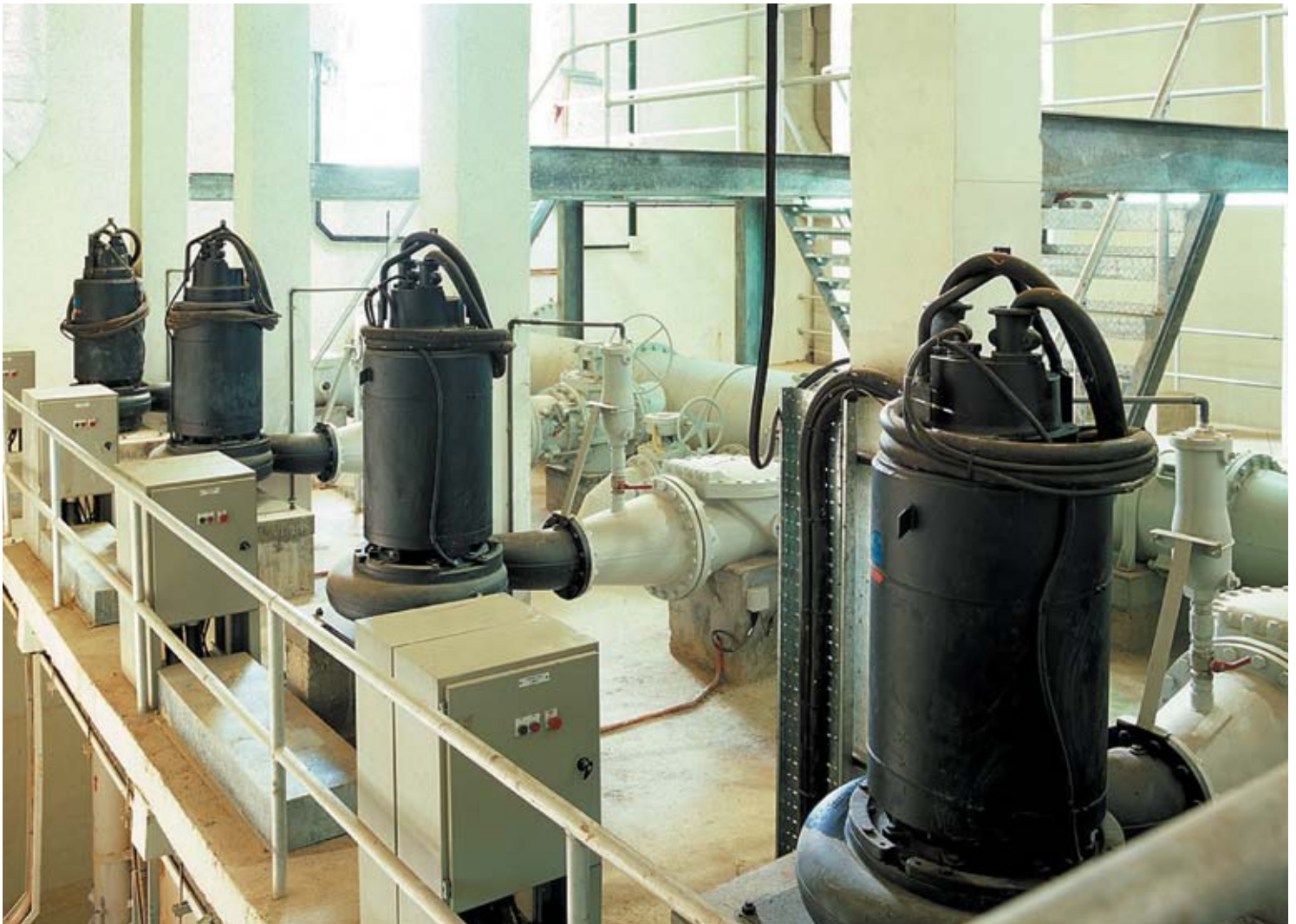
100,000 PE Sewage Pumping Station PS6
