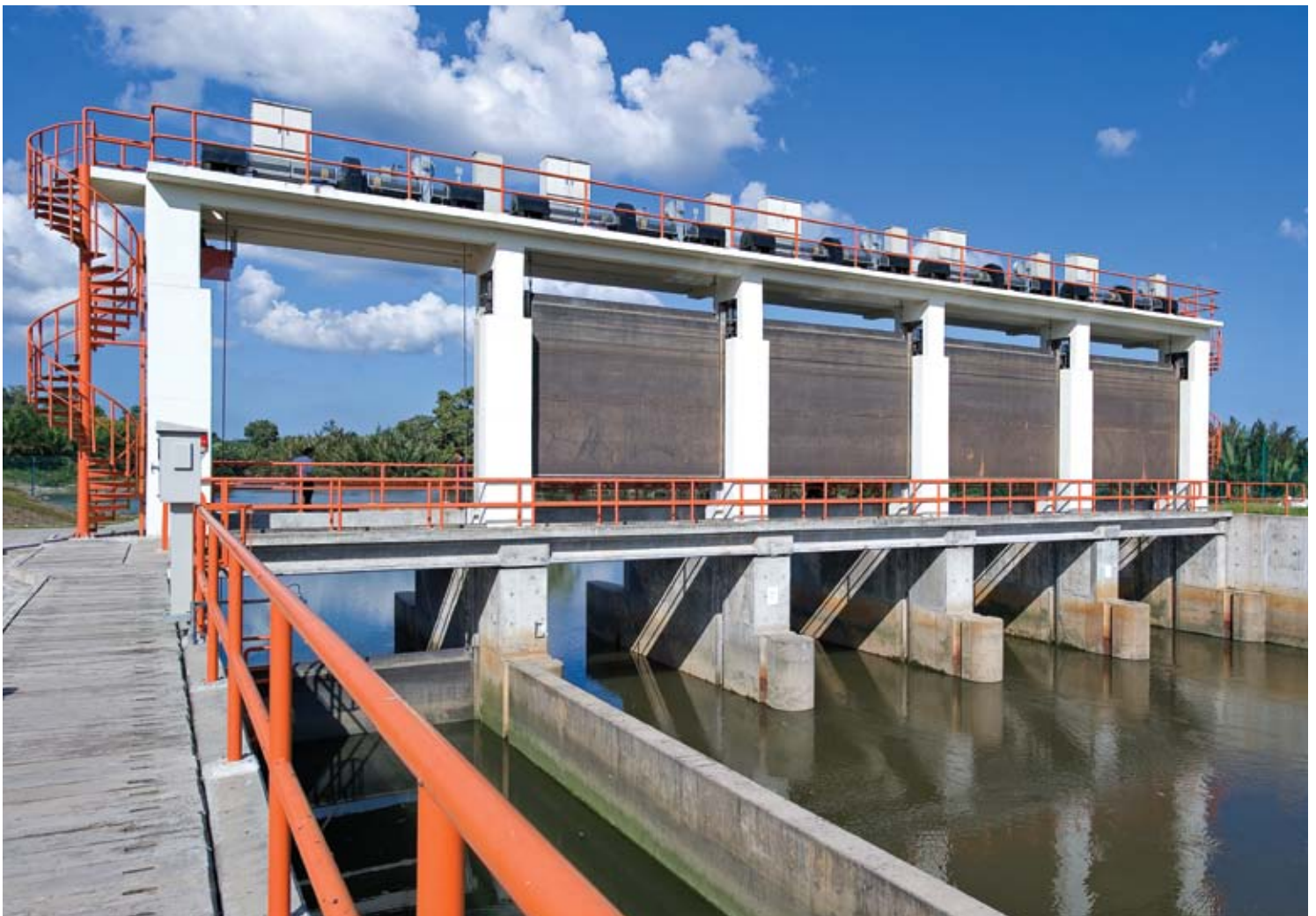
Sandakan River Gates
